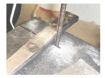
With the bags all eyeballed and in proper position it's time for the hard work-- cutting up the struts. I am sawing it off well before the forward fender bolt hole where the bag will mount. You'll see why in a minute. The strut is just starting to bend up (outward when on the bike) where I am cutting it so the piece I will be left with will be straight.
