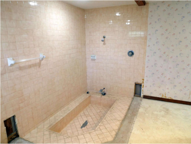
The "pony" or stub wall is ripped out. I thought I got all the mold, but there is more to come.
