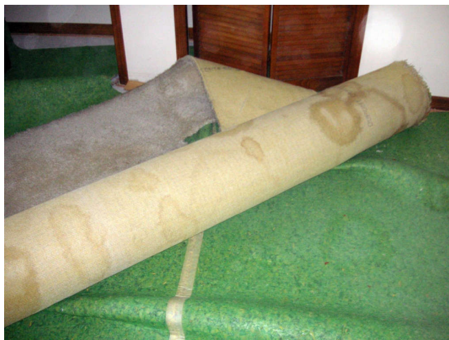
More pee stains on the bedroom carpet. The green is the underlayment mat.
