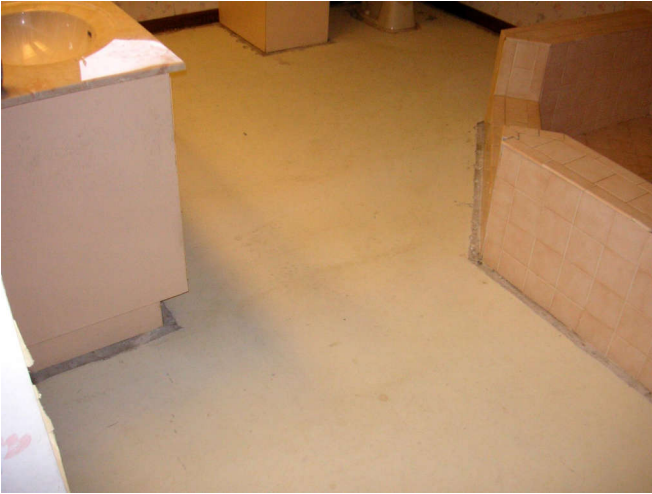
Acetone took the carpet glue off the floor and left it ready for tile.
