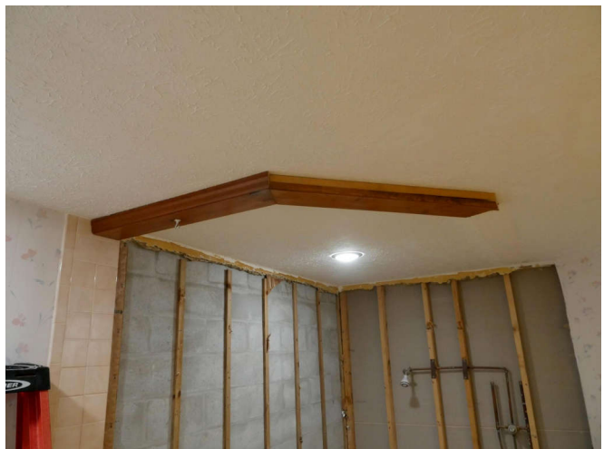
The faux beam on the ceiling gets ripped out.
