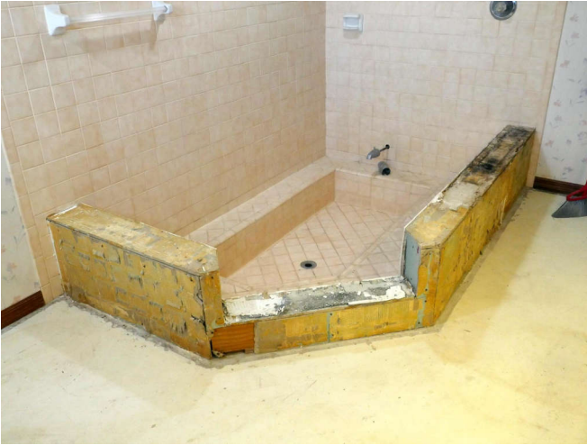
Since the idiots used mastic on the tile, the tiles were easy to pop off the stub wall.
