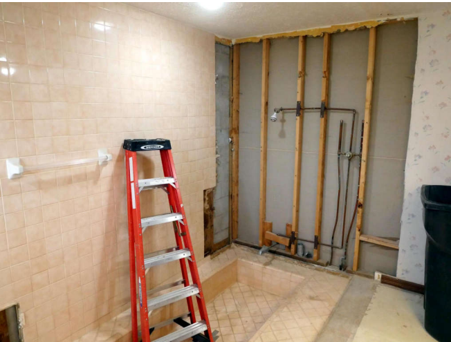
Pulling off the long wall.
