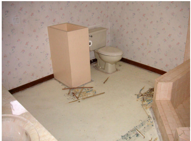
The carpet nail-strips scrapped off.
