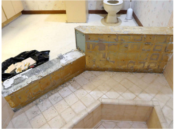
The tiles all held with mastic. Use thinset folks, mastic melts with water.
