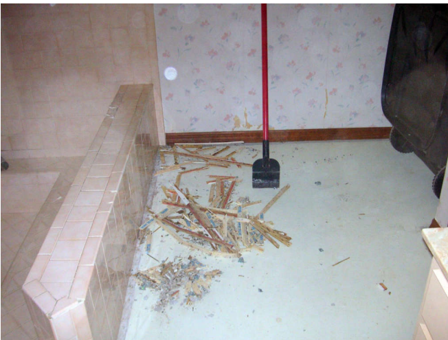
The carpet nail strips scrapped up by the hand tool lent to me by a neighbor.
