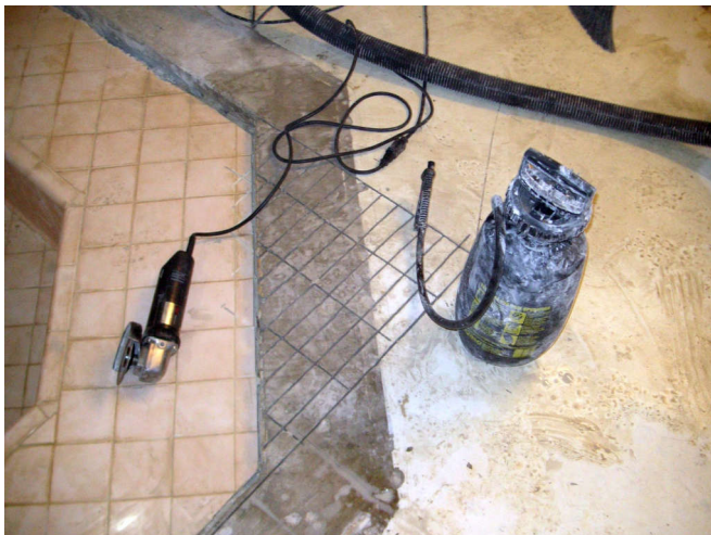
I used a 4-inch grinder with a diamond blade to undercut the blocks where I could reach them.
