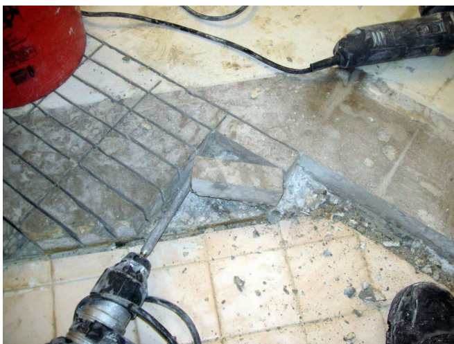
I cleaned up the edge where a partition wall will go, and now break out the rest.
