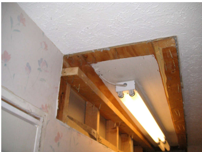
The upper rear frame rail was nailed to the plywood, a hammer helped coax it out.
