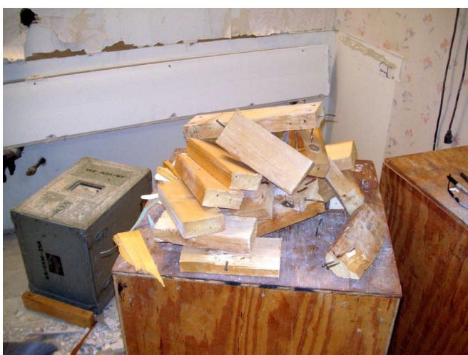
Lots of little cripple studs, but nice dry wood that did not weigh a lot in the garbage can.
