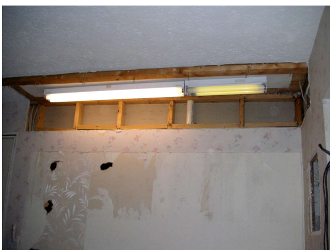
I had to leave the front top frame rail in since it opened to the attic. Same for the plywood.
