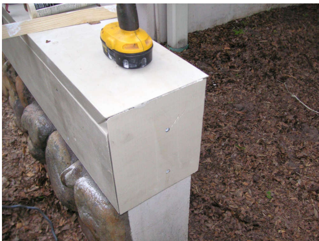
The end cap goes in properly and looks good.
