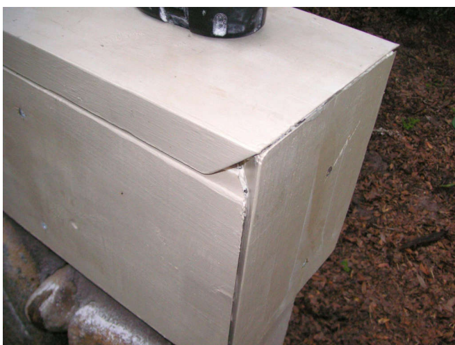
The way I cut the lumber leaves this little hole in the corner. It was better than the way it was originally , with a diagonal cut on the top board.
