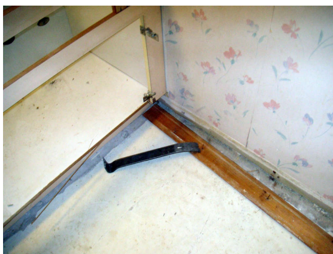
The vanity would not move on one side. This baseboard was keeping it from moving.
