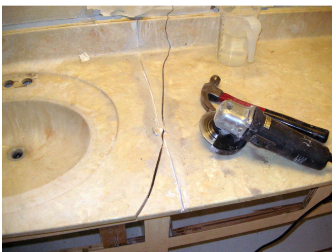
A hammer broke the counter-top in half with one whack. The grinding a slot was a waste.
