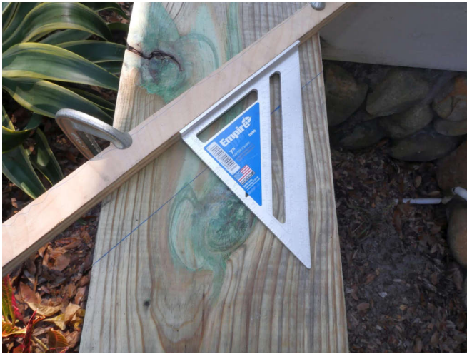
The setup for the angle cut.
