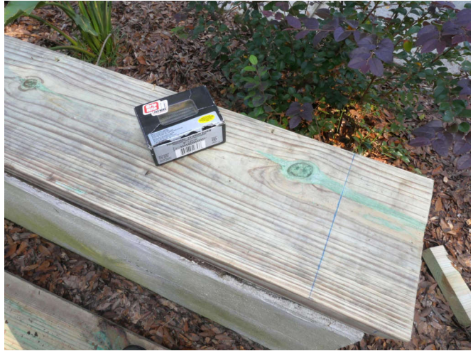
The cut marked, and the 3-inch exterior screws I used to hold the top and front piece together.
