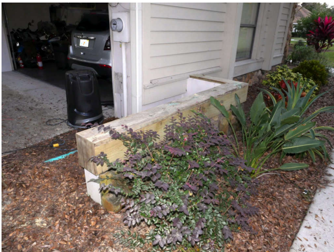
The wall screwed together, but just setting on the concrete. I will anchor it after paint.
