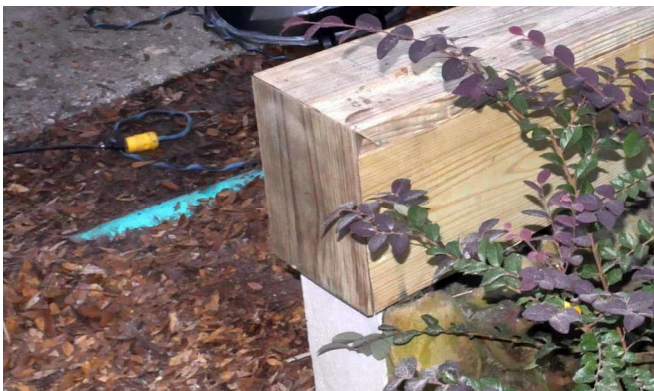
There is a little triangular hole in the corner. I prefer this to cutting a diagonal across the top where water can enter and rot the wood.
