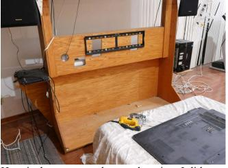
Here is the mount at the new location. I did a lot of figuring to reduce the gap between the screens. A jigsaw enlarged the plywood holes.
