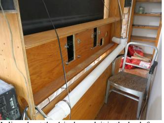
I slipped out the 4-inch conduit in the back for access to the mounting screws and cables.
