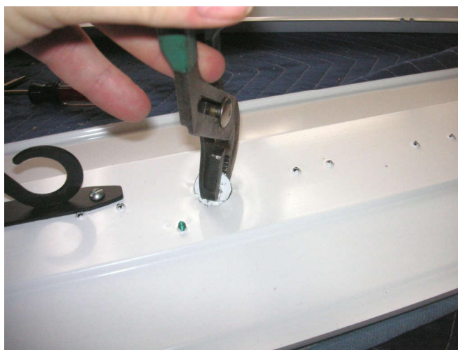
I run a cord from a knock-out on the back.
