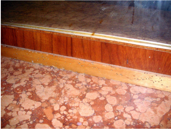
There are worm holes in some of the wood, I assume this is just fake antiquing.
