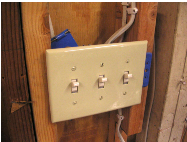
I added a plate for a switch box in the garage.
