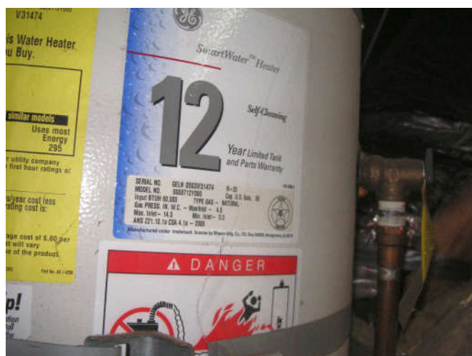
Here is the GE 50-gallon 12-year water heater. Note it has the earthquake strap around it.
