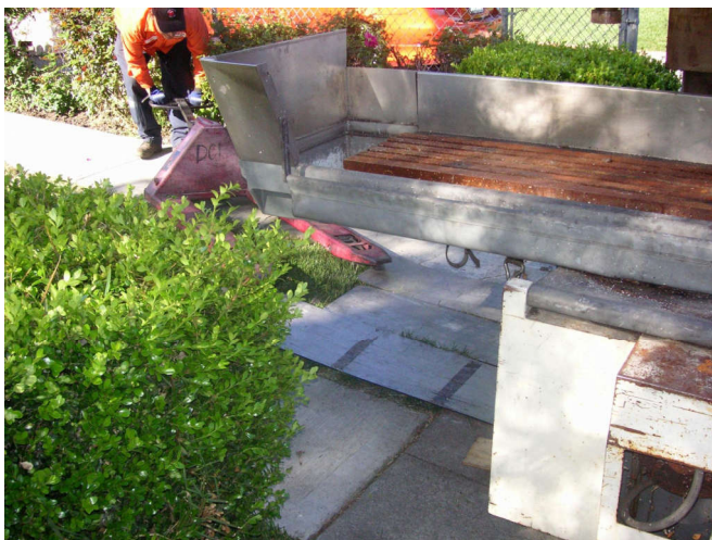
They used the pallet jack to angle the steel plate.
