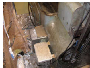
It had an inductor for noise and brake resistors.
