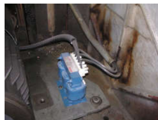
It had an inductor for noise and brake resistors.
