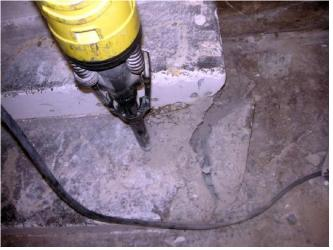
Here is the jackhammer bit doing its thing on the bottom step. It broke apart in less than an hour. It was a great feeling.
