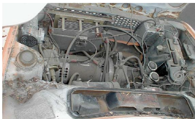
The engine compartment is not as crowded as with a gas engine. That motor and controller are heavy though. Engines are bulky but mostly hollow. This is the motor compartment now.
