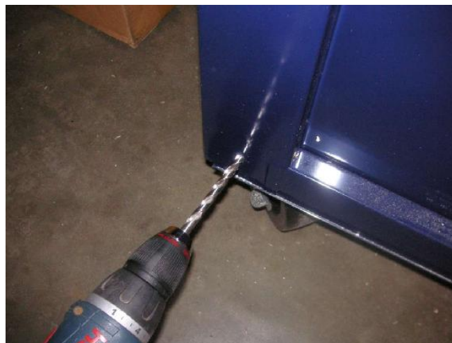
Now enlarge the hole for the 5/16th bolts.
